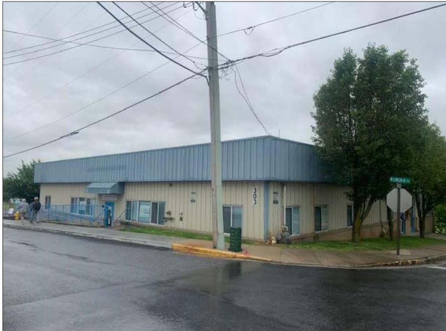
SUBJECT PROPERTY NORTH AND WEST FAÇADES
