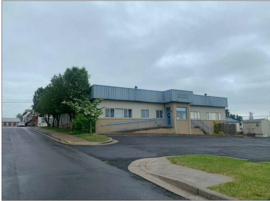
BUILDING REAR – SOUTH FACADE
